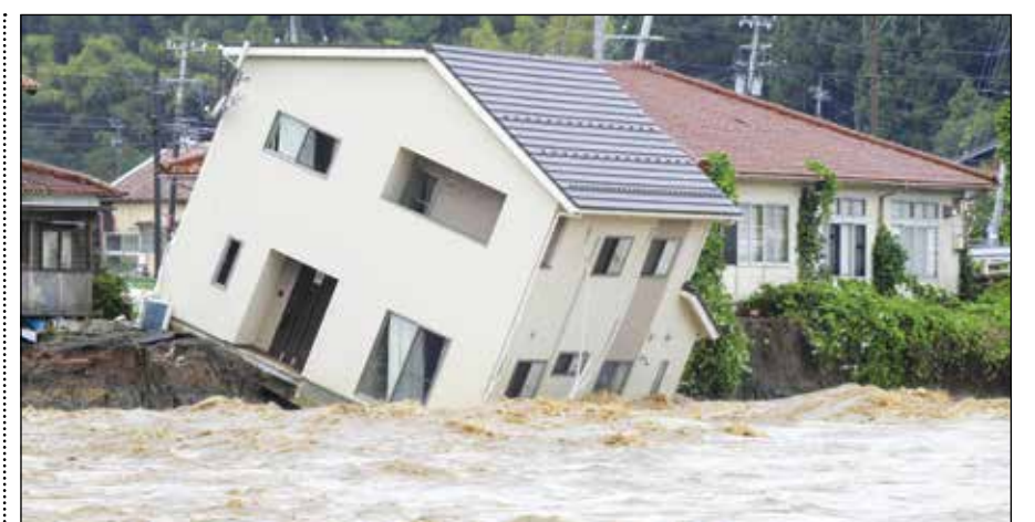
A house leans as a swollen river undermines the ground in Suzu in Japan.
