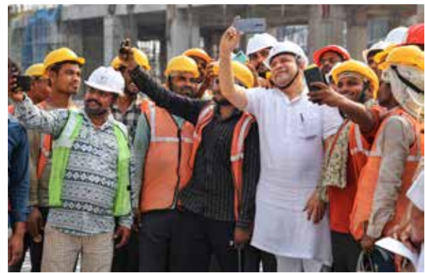
Union Railway Minister Ashwini Vaishnaw takes selfie with workers during an inspection visit of the under-construction Gandhinagar Railway Station in Jaipur on Tuesday. Pic: PTI
