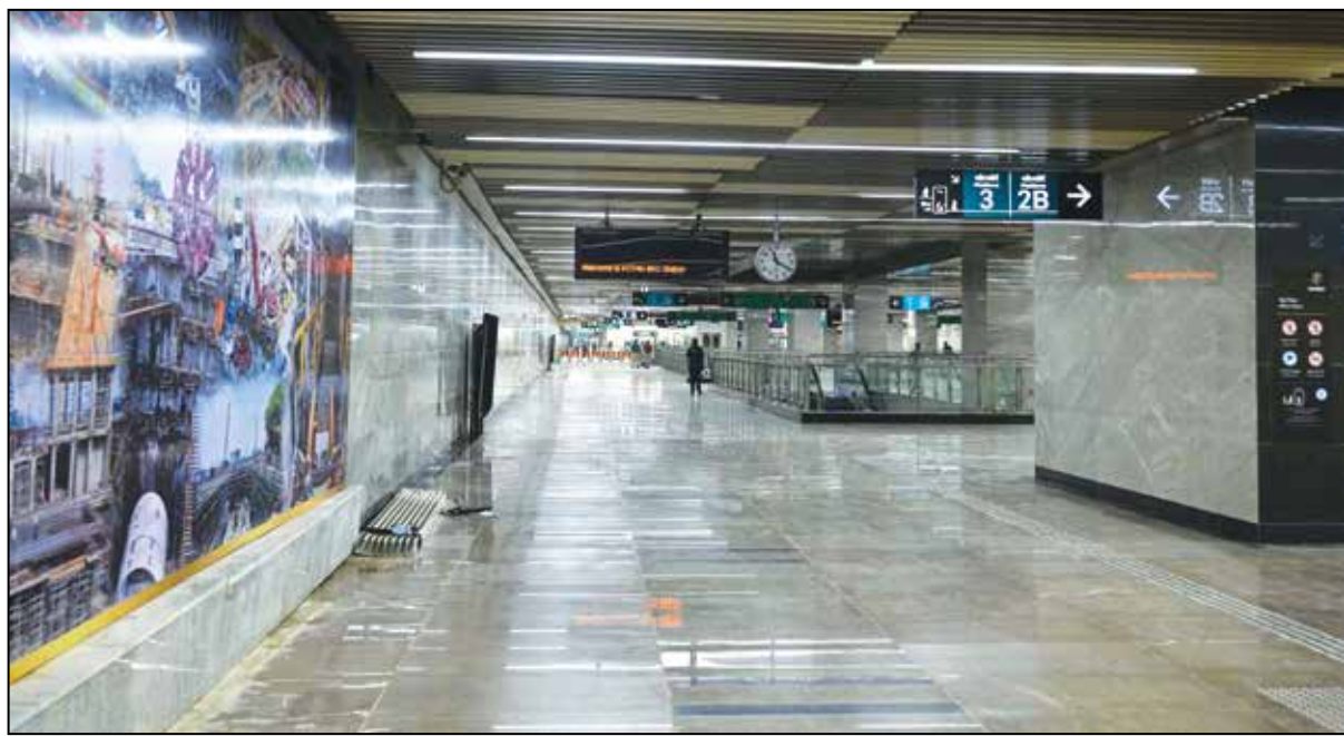
The underground metro is getting ready for the services. Around 93 per cent of the work is completed. The Prime Minister Narendra Modi is likely to inaugurate the first phase in October. Pic: Bhushan Koyande
