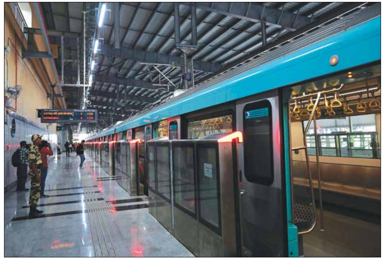
The underground metro is getting ready for the services. Around 93 per cent of the work is completed. The Prime Minister Narendra Modi is likely to inaugurate the first phase in October.
