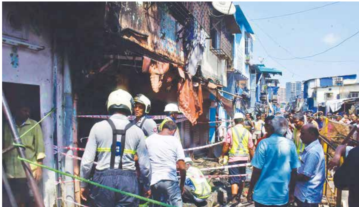
A fire broke out in a double-storey shop-cum-residential structure at Siddharth Colony, Chembur in Mumbai on Sunday.
